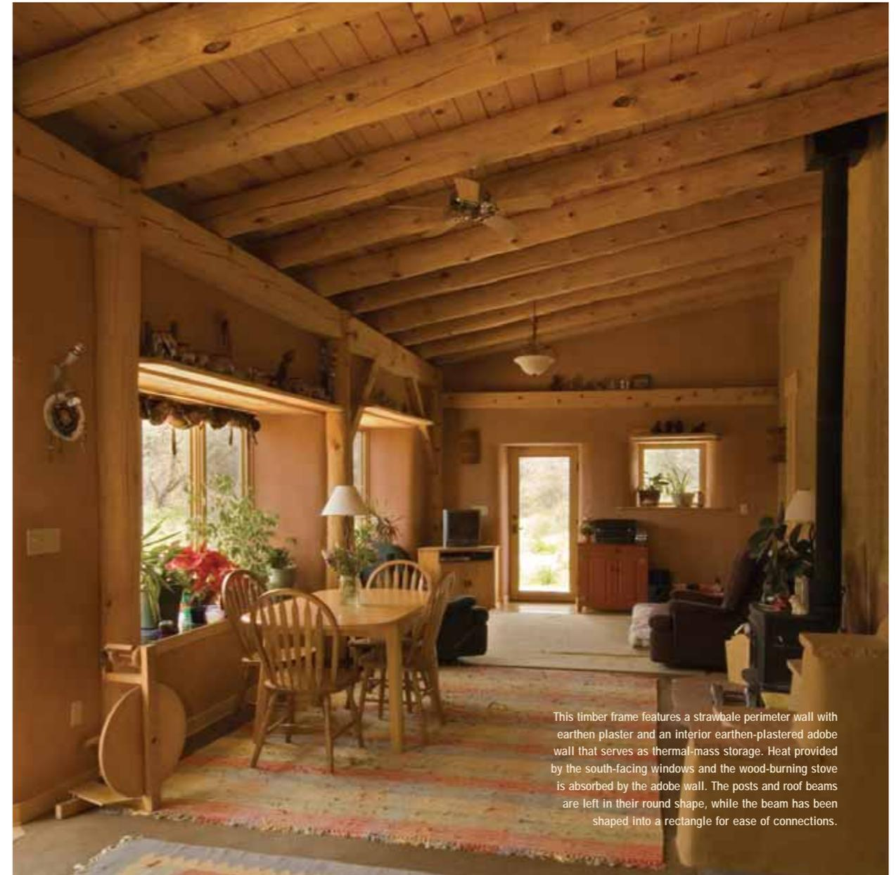
This timber frame features a strawbale perimeter wall with earthen plaster and an interior earthen-plastered adobe wall that serves as thermal-mass storage. Heat provided by the south-facing windows and the wood-burning stove is absorbed by the adobe wall. The posts and roof beams are left in their round shape, while the beam has been shaped into a rectangle for ease of connections.
