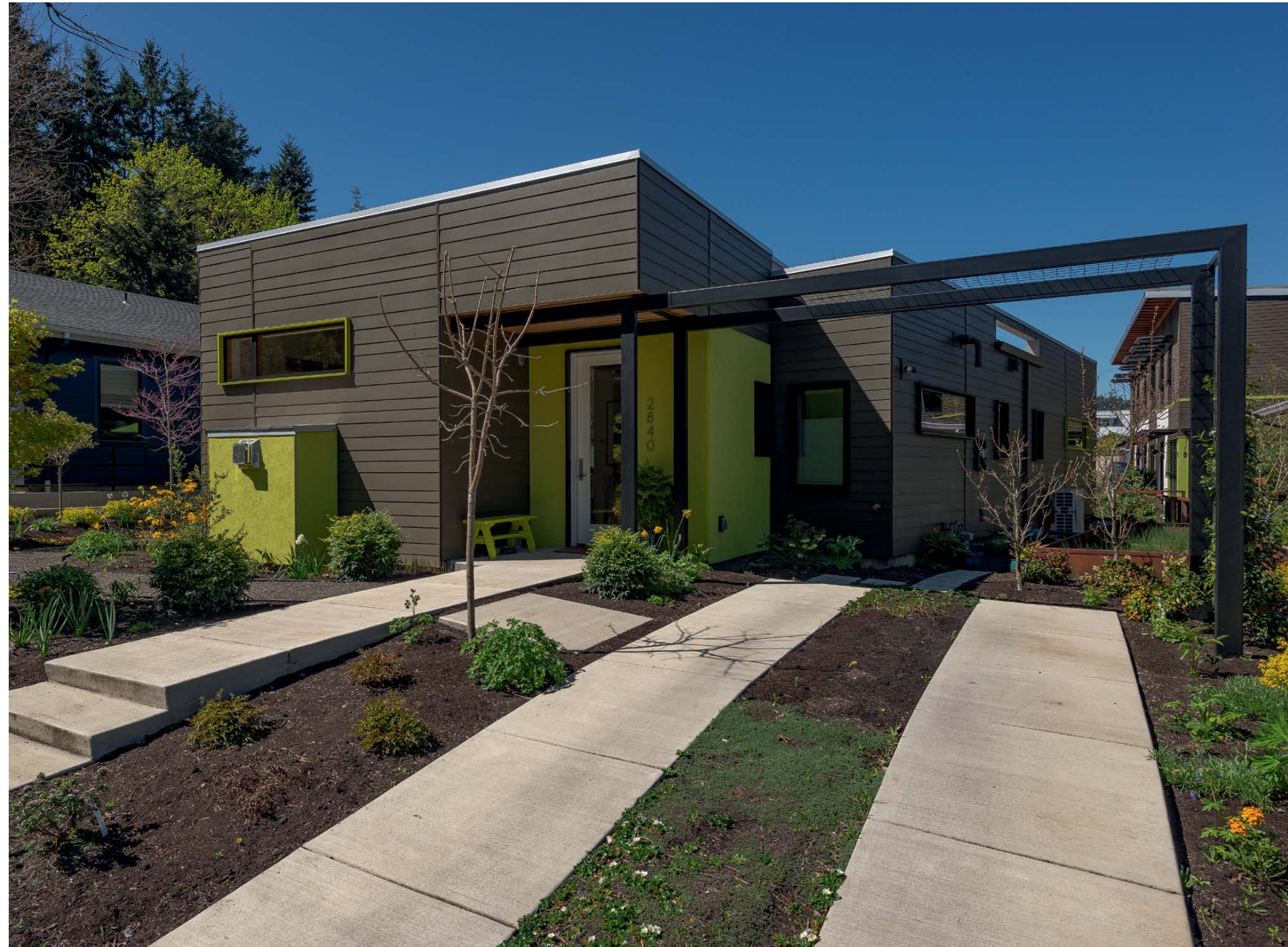
Above: The exterior of the house has fiber cement siding, which is long lasting and low maintenance. (Photo courtesy of Aaron Montoya, www.themontoyacollective.com .)
