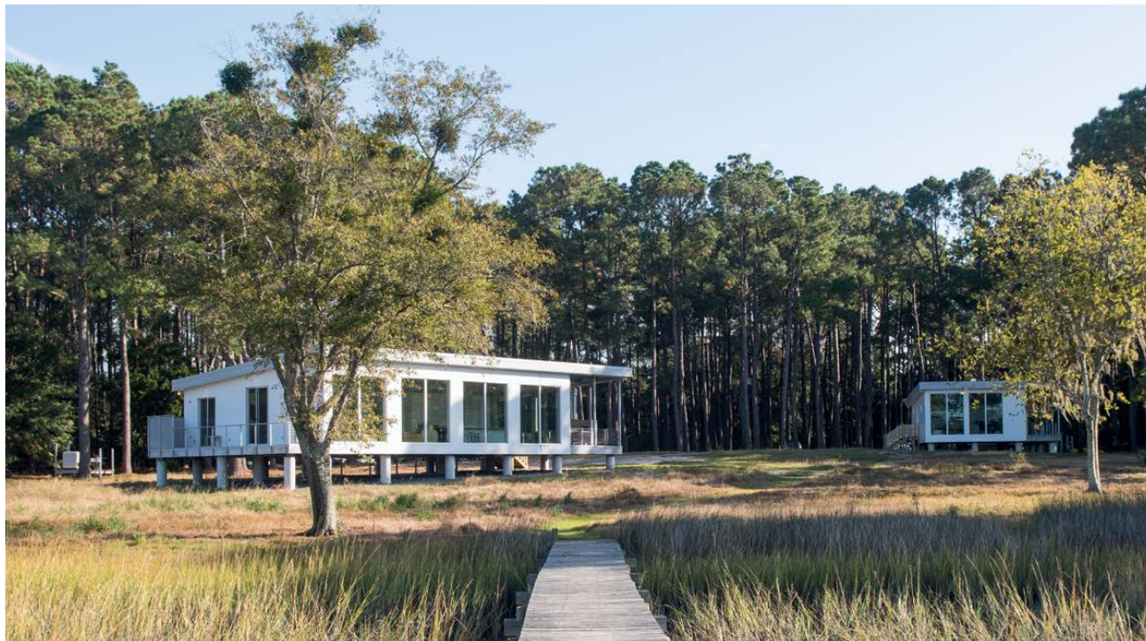
Above: The main house is close to the ADU, which is used as a schoolhouse for the couple's three children and a guest house. Both structures are on concrete pilings to keep them above rising water.
